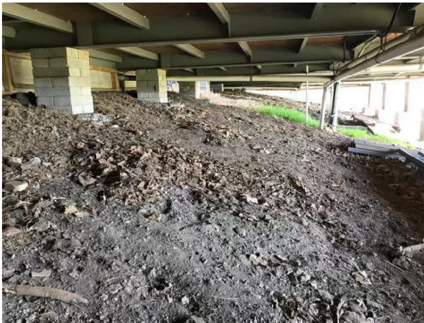
Photograph 2; Evidence of filling beneath and surrounding a demountable building, with surficial demolition rubble and waste visible at surface
